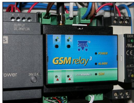
GSM relay to enable remote control via cellphone.
