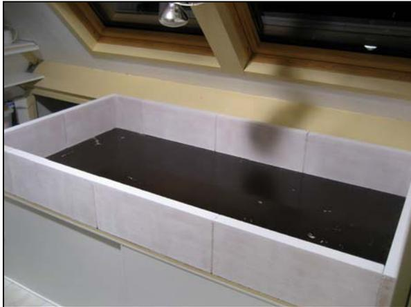
The juvenile enclosures were built of Ytong blocks that were glued to a water tight chipboard plate.
