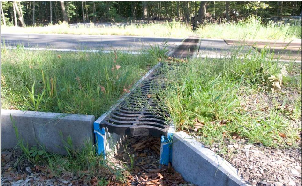
**Figure 7.2** Concrete, mesh-covered gutter to allow herpetofauna to cross a tar road near Hilversum, Netherlands. The mesh ensures that the gutter will have a non-threatening microclimate for fauna. Note the concrete blocks that guide fauna to the gutter entrance.
